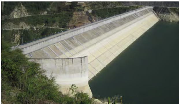
Fig. 1. General view of the Malutang II CFRD.
